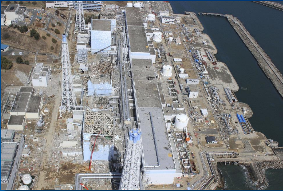
Fukushima Daiichi Nuclear Power Plants on March 24, 2011 (Photo Courtesy of TEPCO)
